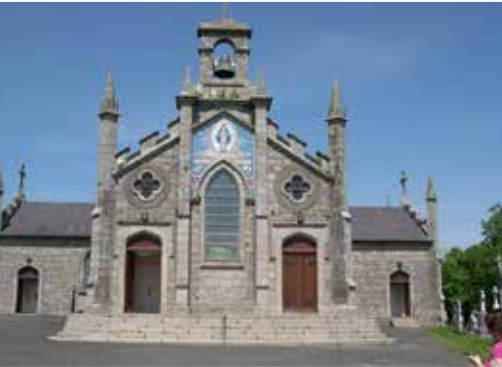
Newtown Church – exterior (above) interior (below)
